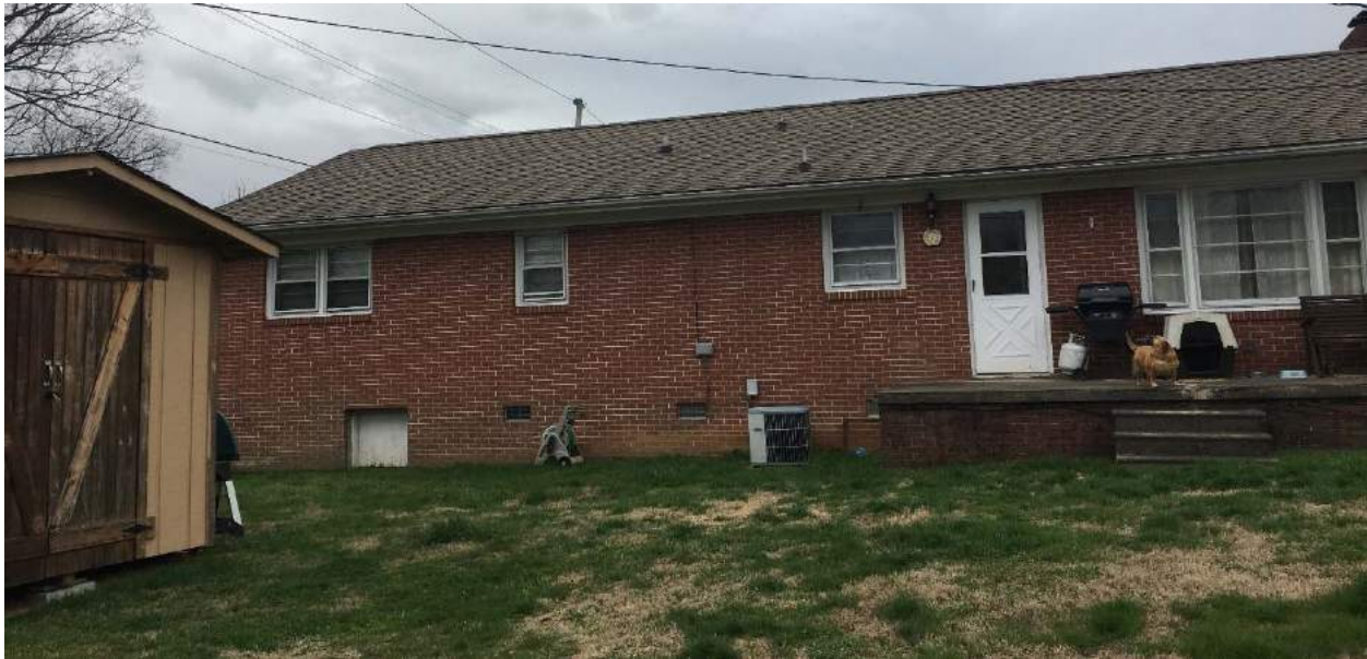
Parsonage, rear view to the south
