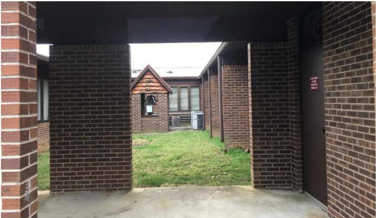
West Hendersonville Baptist Church, interior courtyard, view to east
