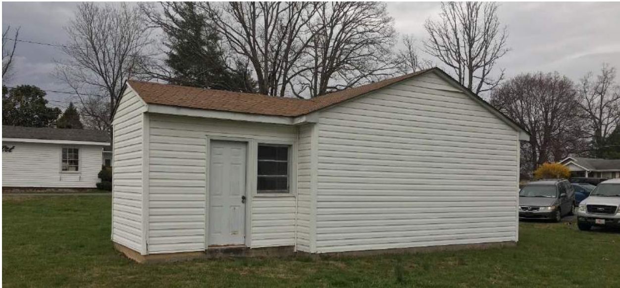
Storage Building, west elevation, view to east
