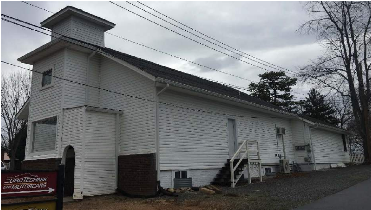
309 White Street, oblique front view to northwest
