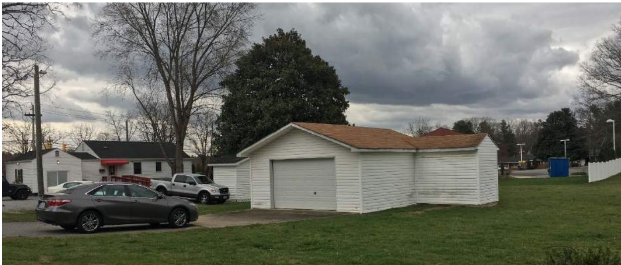
Storage Building, oblique front view to southeast
