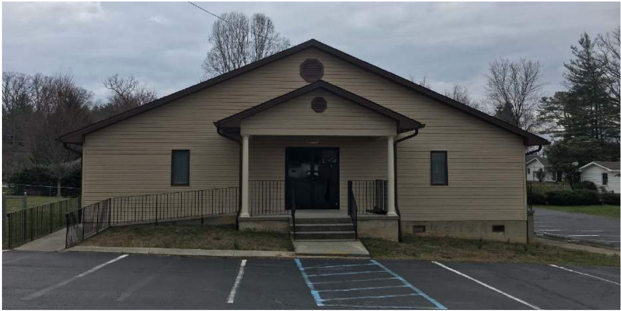
Fellowship Hall, façade, view to north
