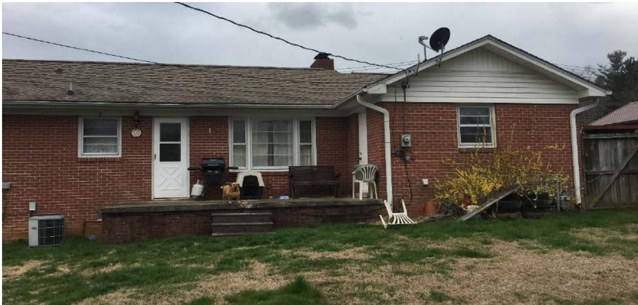
Parsonage, rear view to the south
