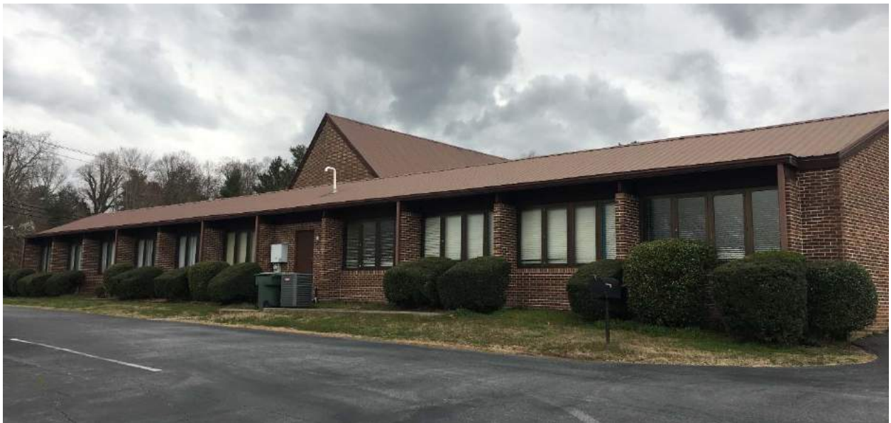
West Hendersonville Baptist Church, oblique east elevation view to the southwest
