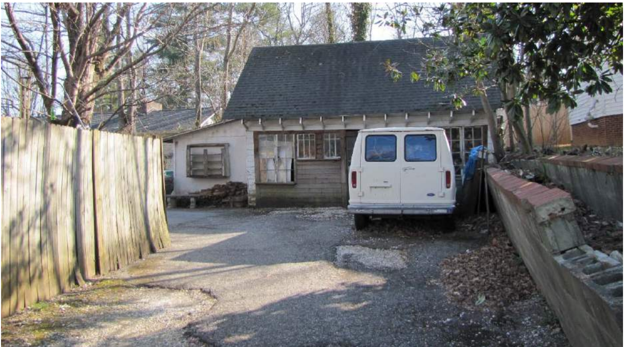
Outbuilding, north elevation, view to the south
