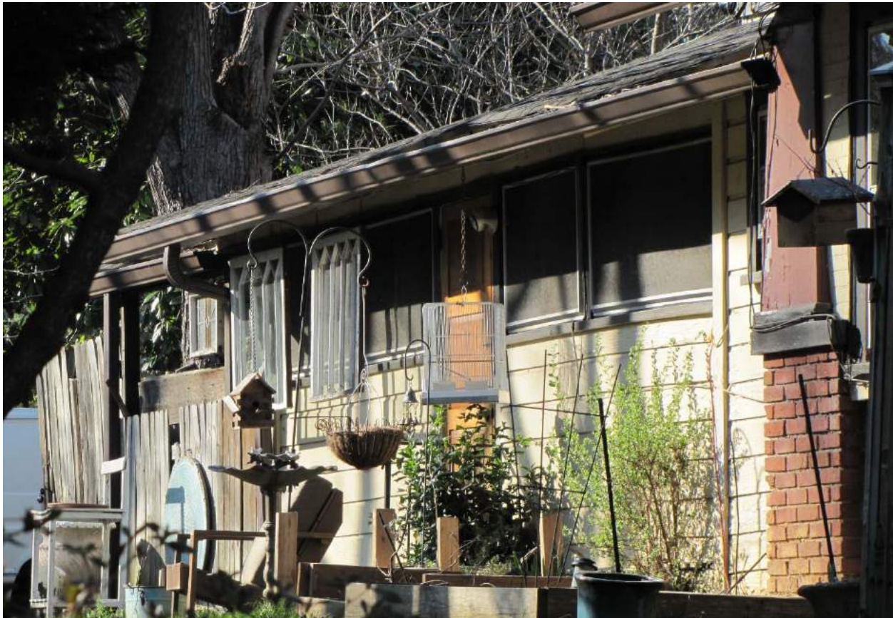
Poplar Terrace House, south elevation sleeping porch, view to the northwest
