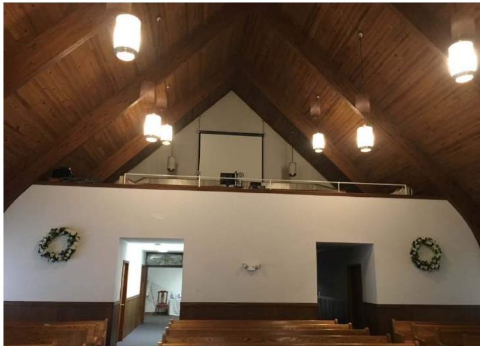
West Hendersonville Baptist Church, sanctuary gallery, facing east
