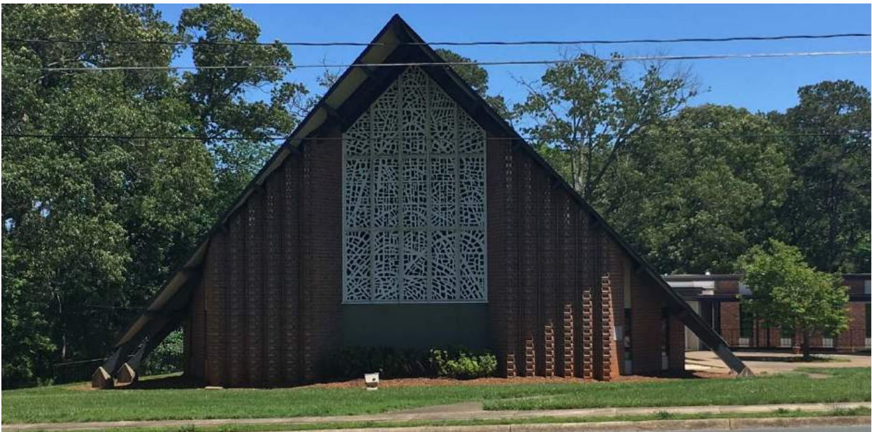
Highland Methodist Church, 1020 12 th Street Place NE, Hickory, NC. Photos by Author April 2017.
