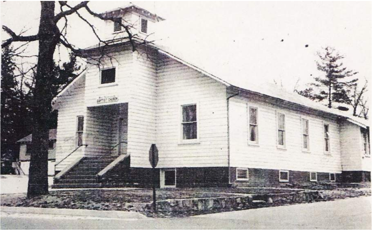
Ca. 1940's photograph of the church location at 309 White Street. 50
