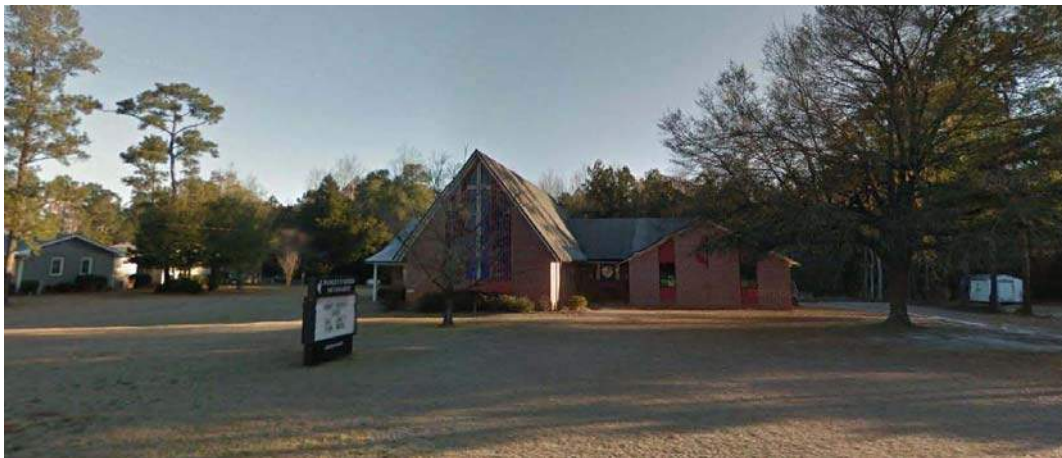
Wesley United Methodist Church (CB0190), 104 NC Hwy 87 Columbus County, NC. Google Earth Photo.
