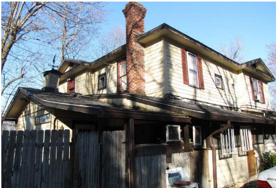
Poplar Terrace House, oblique rear view to northeast
